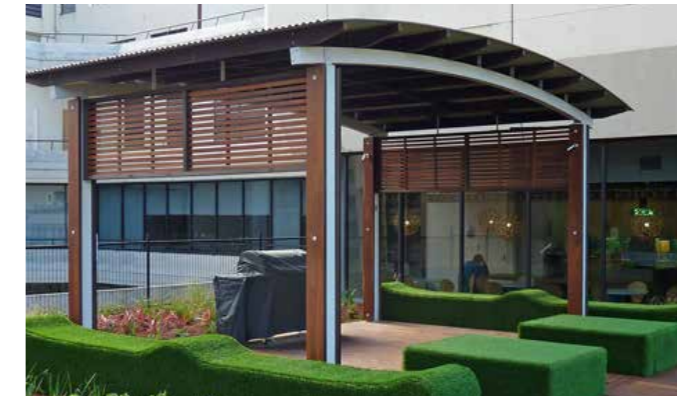
Customised landmark structure note the steel posts faced with timber and prominent steel bolts, create a durable structure with a domestic aesthetic
